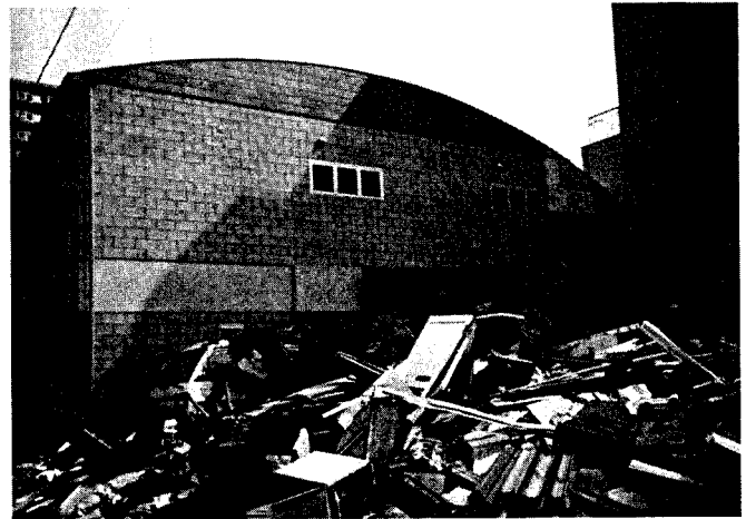
Fig. 8. Undamaged small reinforced masonry building located in Kobe (from Japanese Society for the Promotion of RM Buildings).
