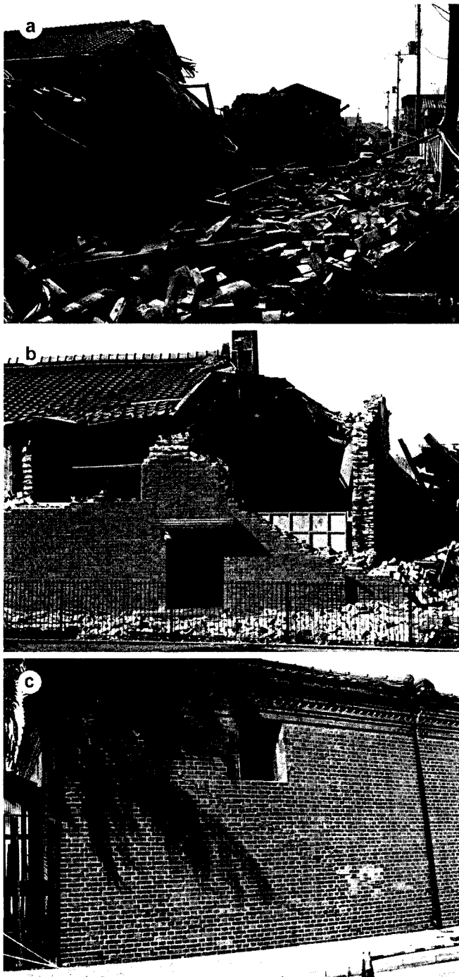
Fig. 3. Collapsed unreinforced brick masonry buildings of a sake-distillery: (a) global view of rubble blocking a street, and showing type of masonry units; (b) walls partly collapsed in out-of-plane manner; (c) wall with visible in-plane cracking.
