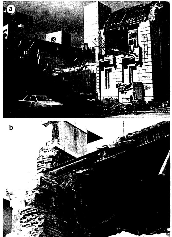
Fig. 4. Severely damaged unreinforced masonry building in downtown Kobe: (a) global view; (b) close-up view of a simply supported gravity structure.
