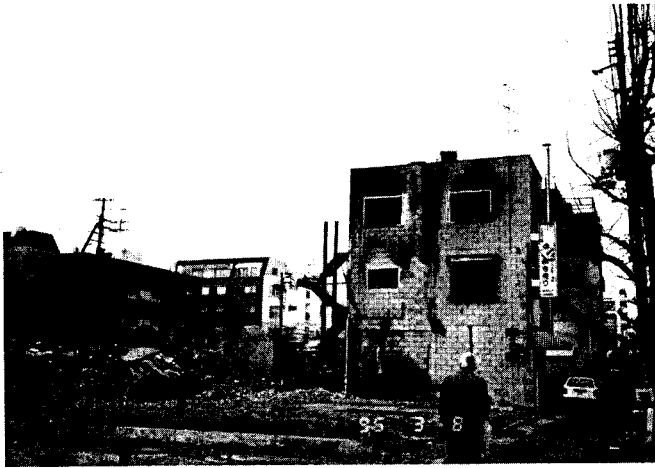
Fig. 9. Undamaged small reinforced masonry building located in Kobe (from Japanese Society for the Promotion of RM Buildings).
